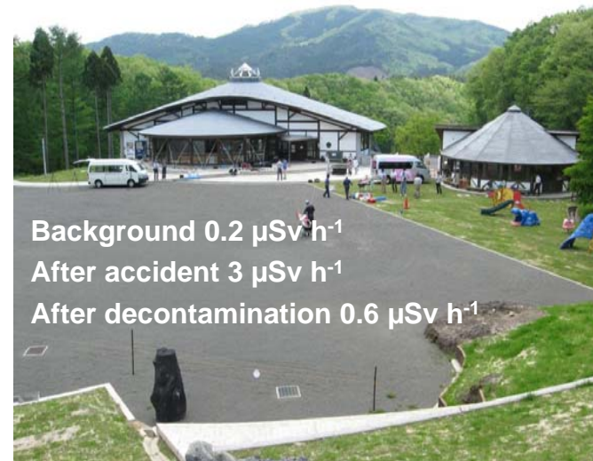
Children's Museum, Date, Japan. Decontamination options used: Pressure washing, shot blasting, sanding/grinding, soil removal
